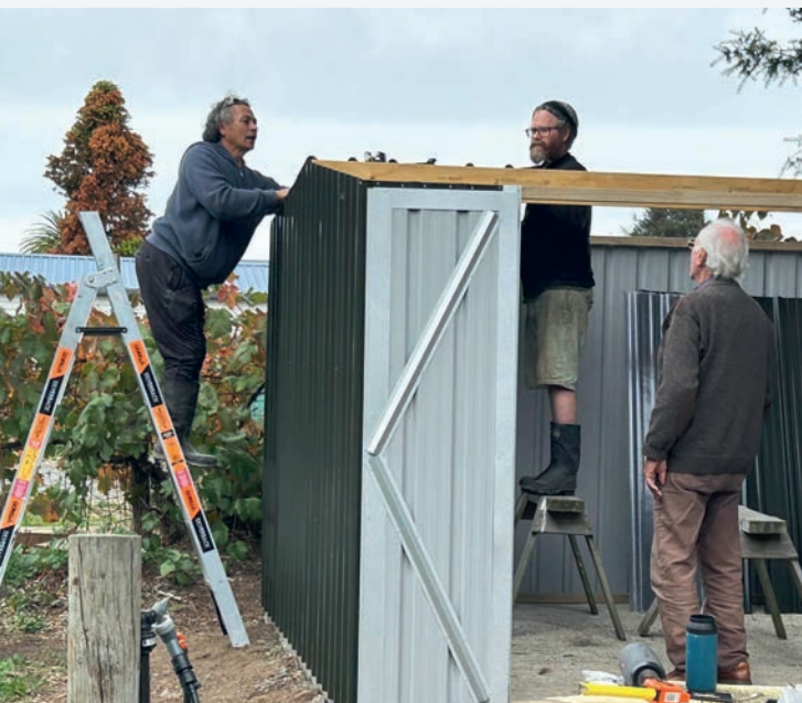
Oxford Street Community Garden shed takes shape.
